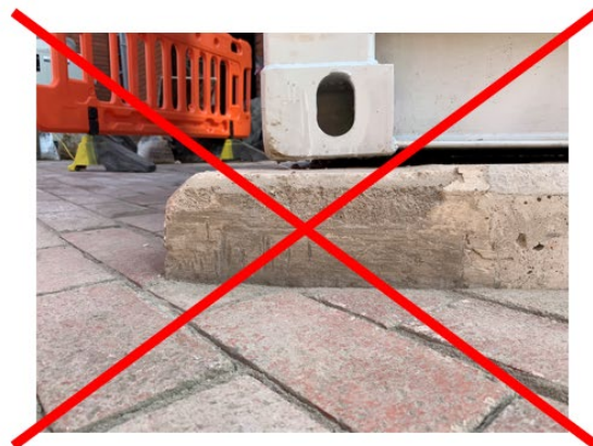
Figure 31: Example of improper - non-levelled placement with hovering corner points
