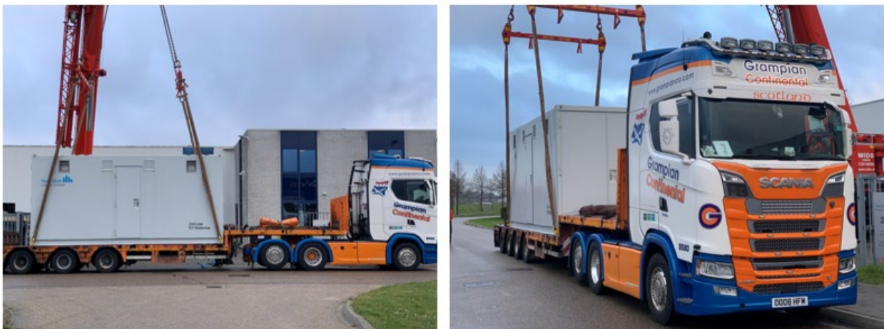
Figure 26: Example of a lifting job
