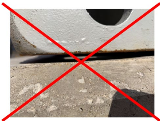
Figure 31: Example of improper - non-levelled placement with hovering corner points
